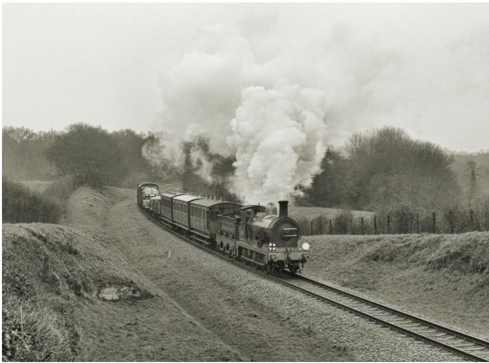
No. 65 at Rock Cutting with a mixed train. Photo: Jon Bowers
