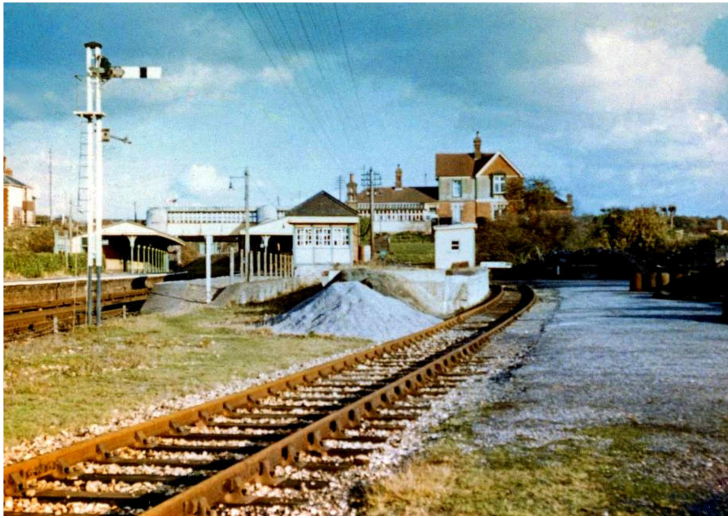
Original shed at Ardingly Station
