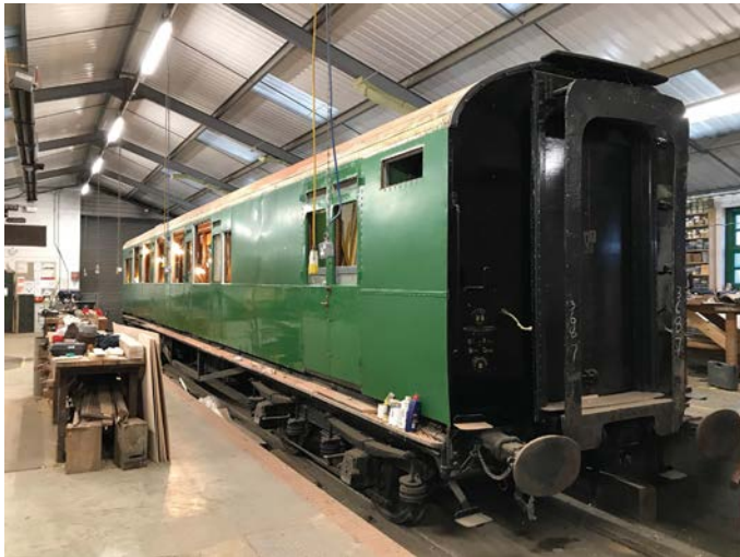
Just before the second lockdown, the east side of Maunsell Hastings Line brake No 3687 received its first undercoat. RICHARD SALMON
