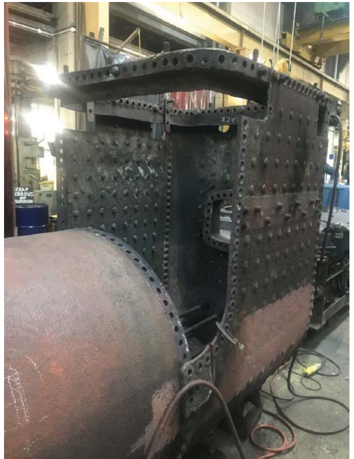
Fenchurch's boiler with the throatplate and inner firebox removed. TOM JAMES
