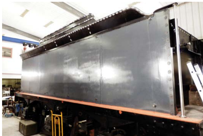
All of the coal rails and their infill pieces plus the beading around the top edge is now all fixed and the heads of the fastenings (seen above as silver spots) will be painted shortly.
