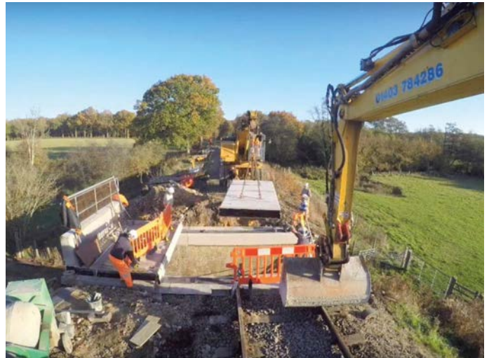
Lifting in the central deck section. ANDY PALMER
