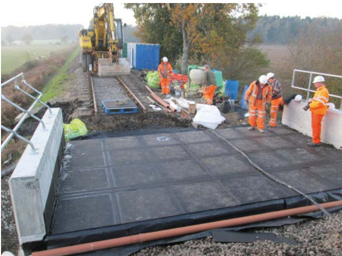
Waterproofed and ready for ballast. TIM CRUMP
