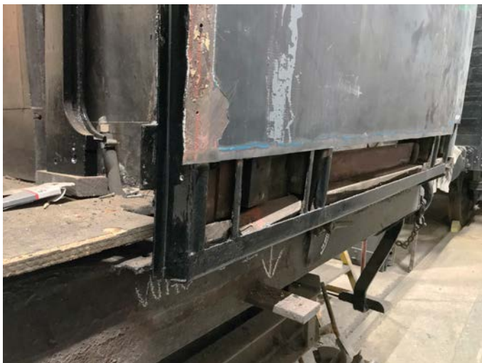
Ex-Bicester Mk.1 TSO, No 4754, is also making progress, with the last structural repairs being to the north end. RICHARD SALMON
