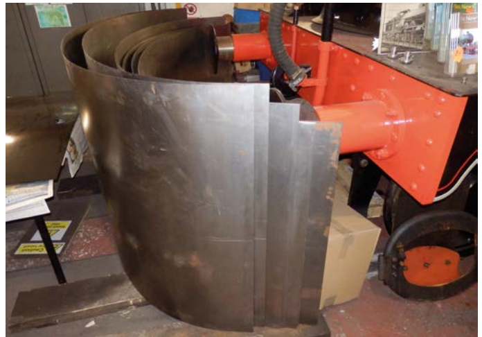
The basic boiler clothing sheets have been laser cut and rolled.
