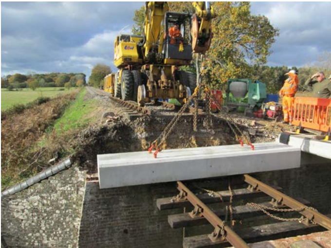
Lifting the main section of sill beam. TIM CRUMP
