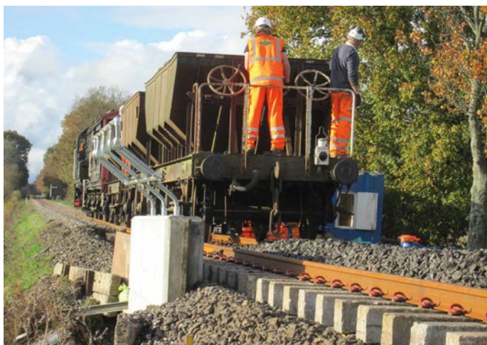
Dropping ballast over the bridge. TIM CRUMP
