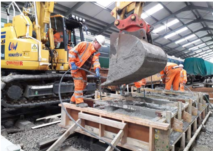
The first deck panel, cast on 18 March 2020. CLIVE WHITCROFT
