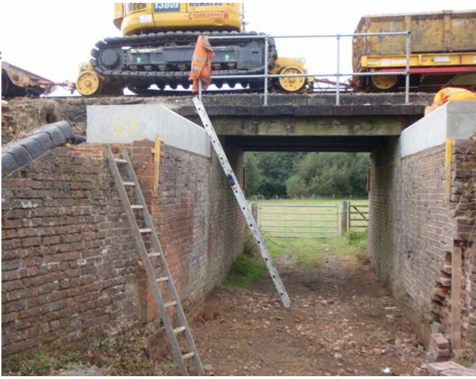
Brickwork required. BRUCE HEALEY
