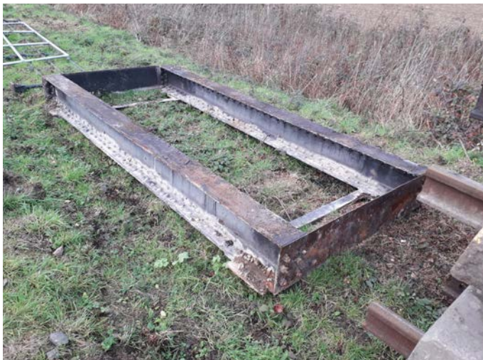
Old and new: Two old wrought iron beams versus 15 new to support each train. BOTH: JON GOFF
