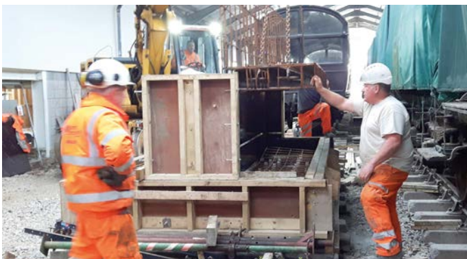
Lifting the I-beams into the parapet sections. CLIVE WHITCROFT
