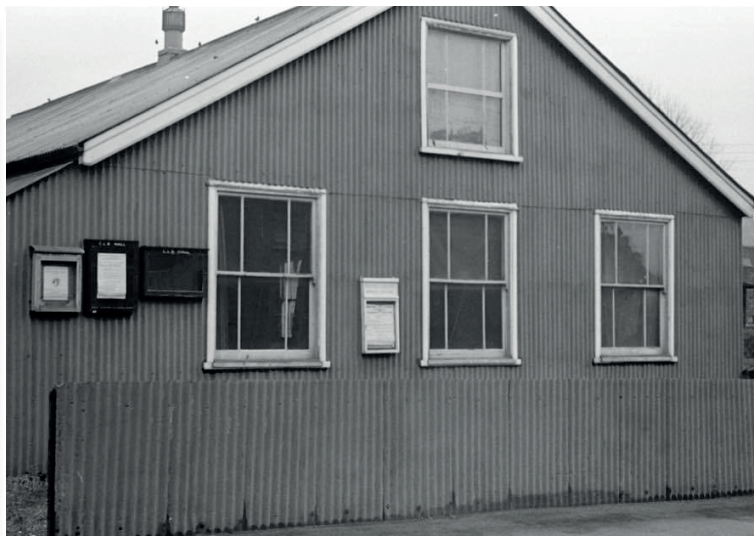
The CLB Hall in Gower Road, Haywards Heath, since demolished. ANDREW ZVIRBULIS
