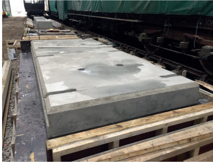
RIGHT: The first castings for redecking Palmers Bridge on lockdown day. ANDY PALMER
