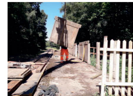
Removing the back panels. JON GOFF
