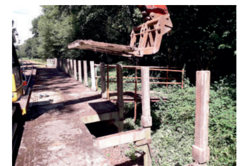
Next came the deck panels. JON GOFF
