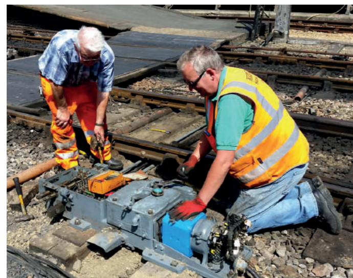
Mick Sargeant, ably assisted by Alan Rogers, adjusting the replacement point machine at Sheffield Park during intolerably hot conditions. MARTIN LAWRENCE
