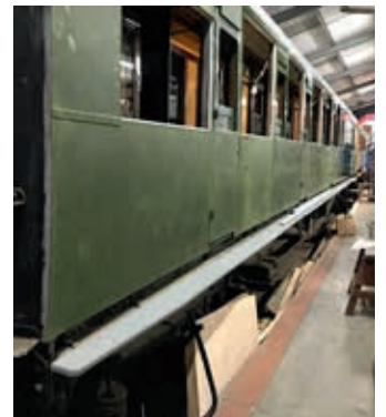
The step boards are machined up and ready to fit on the corridor side of No 3687, which is seen in 'rubbed-down' topcoat.
