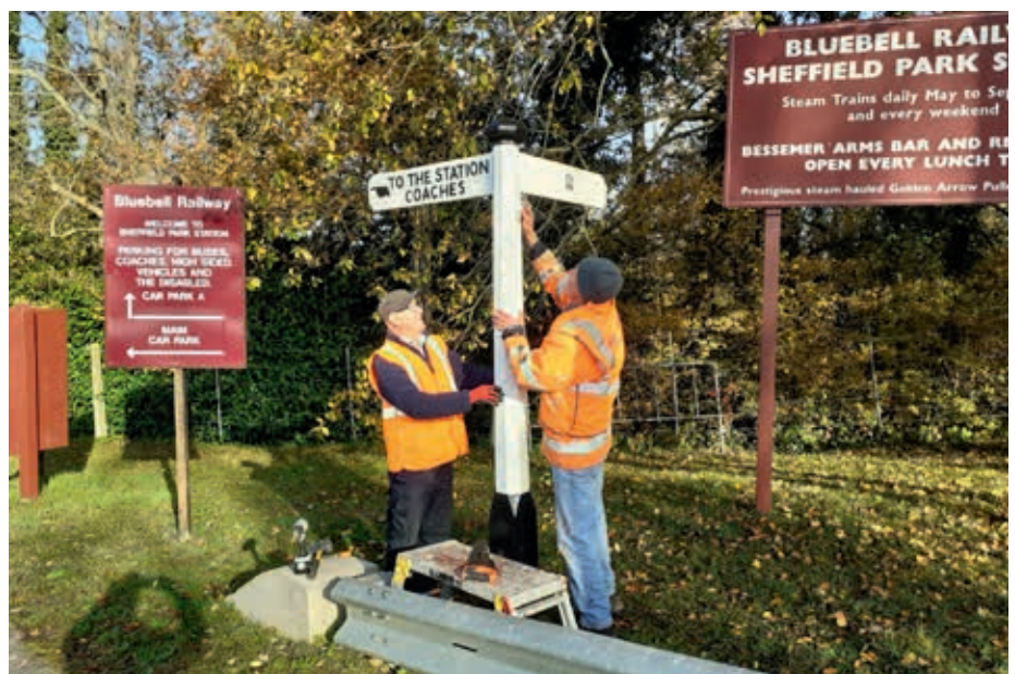
Finishing touches being applied to a repaired finger post.
