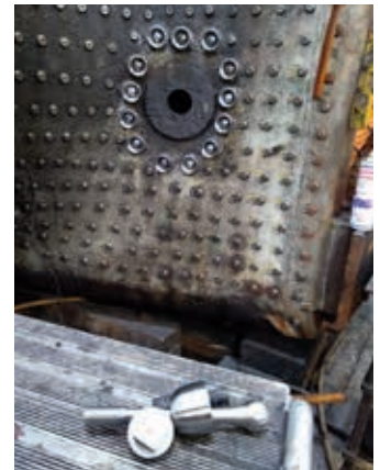
Flexible stays fitted to base of the thermic siphon, with stay in foreground. JOHN FRY
