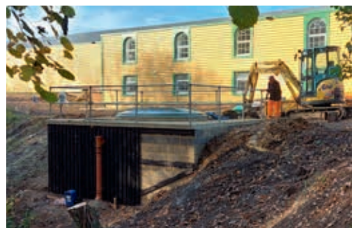
Wooden cladding going in to hide the concrete blockwork. JON GOFF
