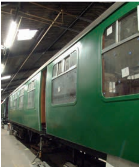
The exterior of ex-Bicester Mk. 1 TSO No 4754 is progressing to undercoat, always a good sign in any project, signifying that the structural repairs are effectively completed.
