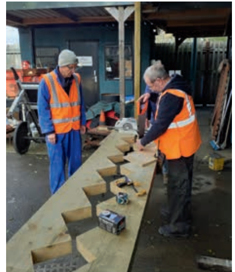
Preparing timber 'stringers' for the replacement staircase in the loco yard.
