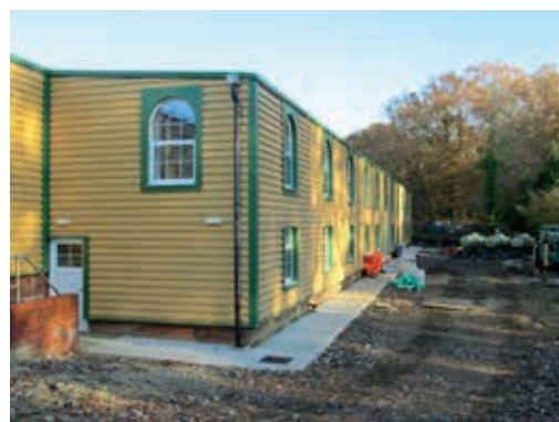
Rear path by the Skills Centre and steps into OP4. TIM CRUMP
