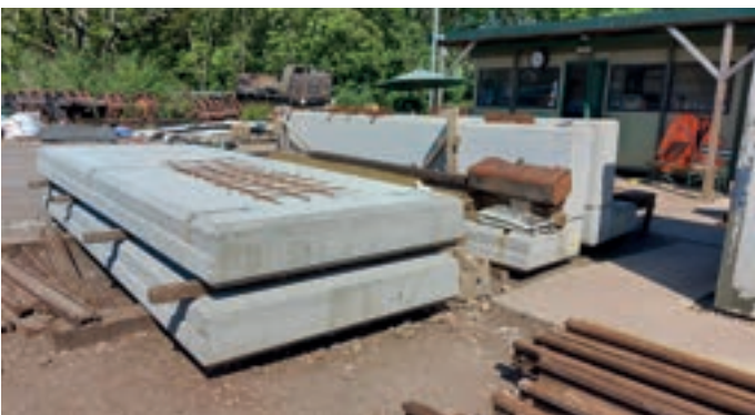
New bridge sections freshly cast for a location on the Ardingly trackbed. JON GOFF
