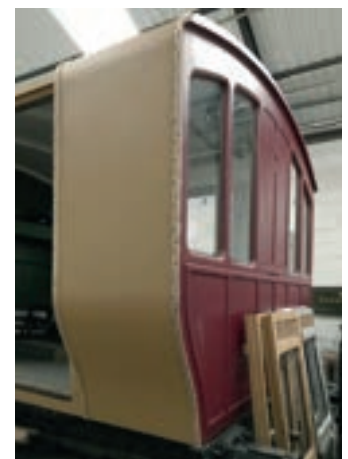
With the glazing of the Stroudley Brake now complete, the finishing touch to the guard's duckets (lookout) has been a complex curved wooden moulding acting as an edging over the steel plate. These plated duckets represent a very early use of metal on carriage exteriors, something which did not become common in the UK for another 40 years.
