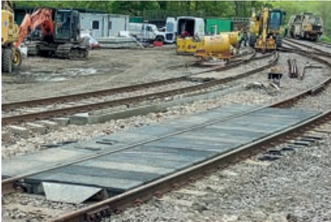
The new vehicle crossing under construction. JON GOFF
