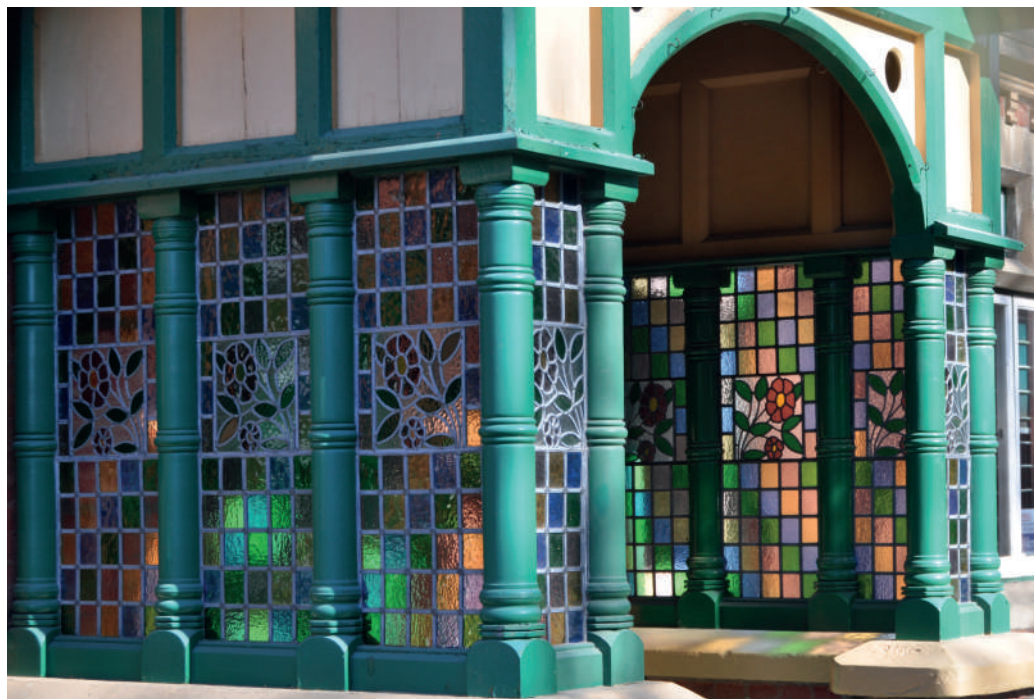
The restored entrance porch.
