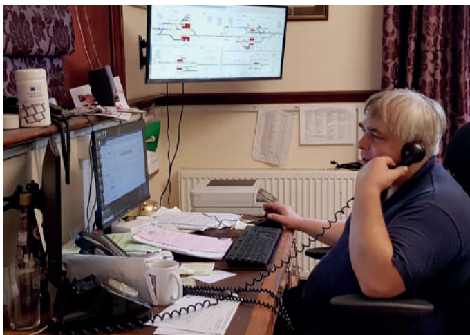
Majview screen installed in the Operations Manager's office.
