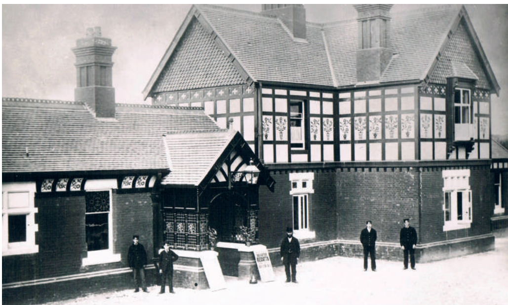
Horsted Keynes station ready for business at the opening year in 1882. The decorative plaster work to the first floor of the station house failed even in LBSCR days and was replaced with a continuation of hanging tiles in the Sussex style. It would not be cost-effective to return this appearance.
