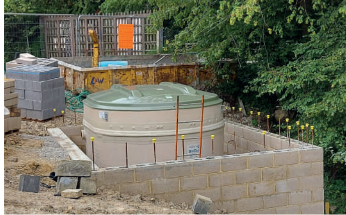
The septic tank in place with retaining wall. JON GOFF
