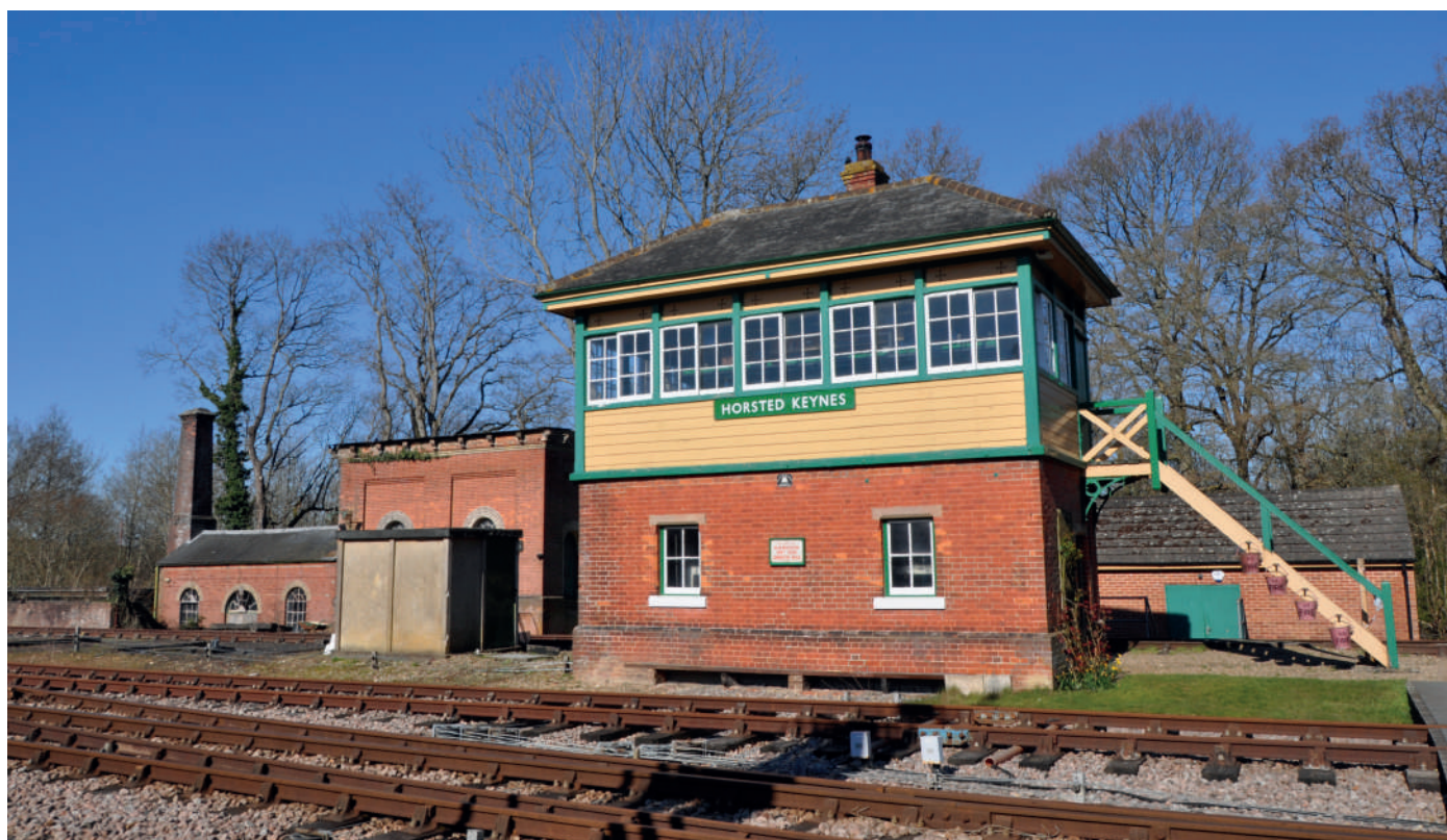
The signal box and adjacent former pump house and water tower are also Grade II Listed. Only the signal box comes under current restoration plans.
