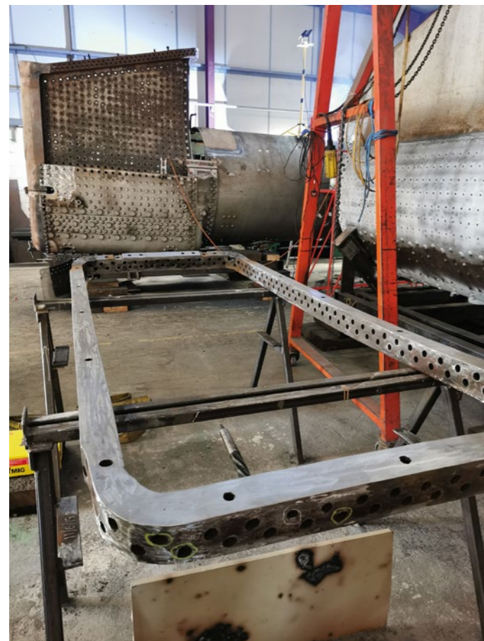
Stowe's foundation ring under repair. HBSS
