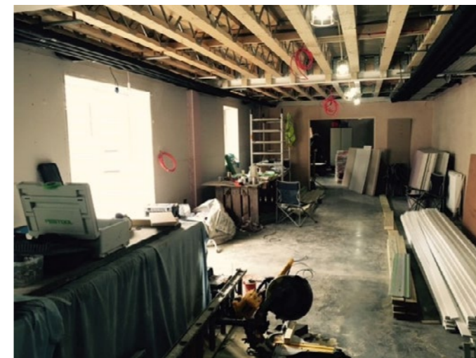
The new trim shop and moquette store on the ground floor.
