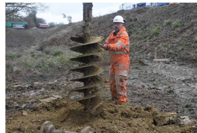
Andy Palmer clears spoil from the auger. JON GOFF
