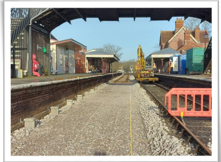
Laying sleepers to the line. Photo: Jon Goff
