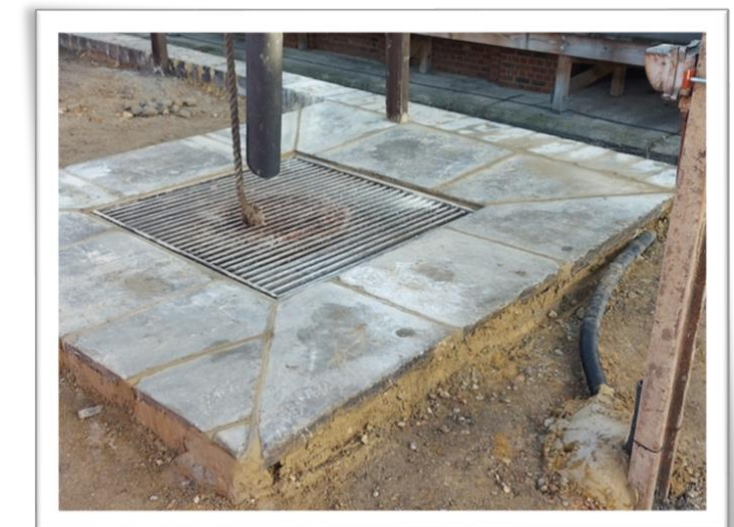
Drain surround replaced. Photo: Jon Goff
