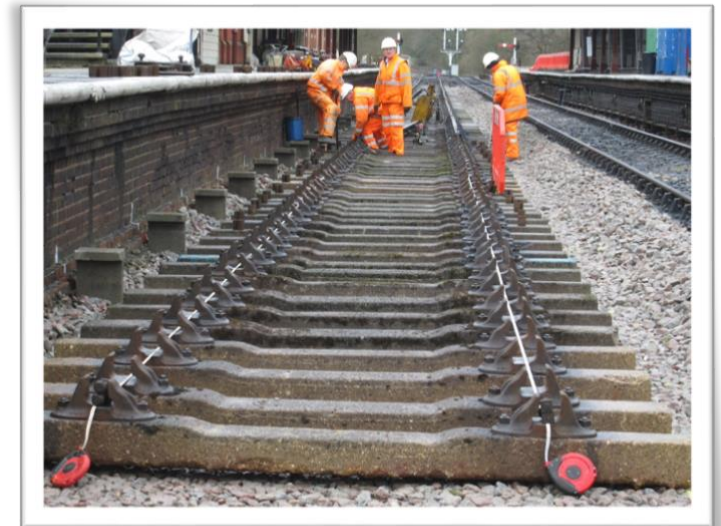
Adjusting the sleeper positions. Photo: Tim Crump
