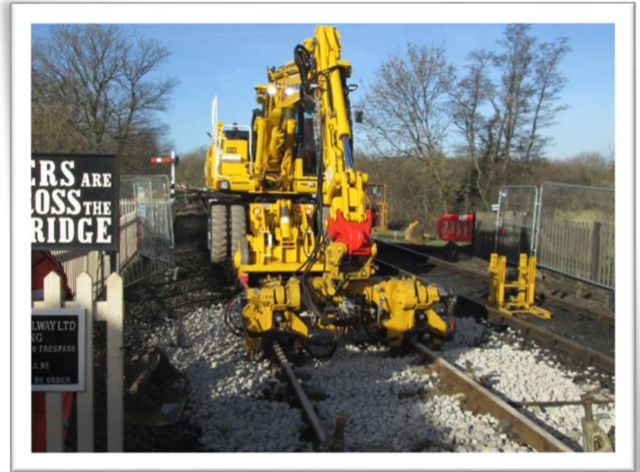
Starting the initial tamp. Photo: Tim Crump
