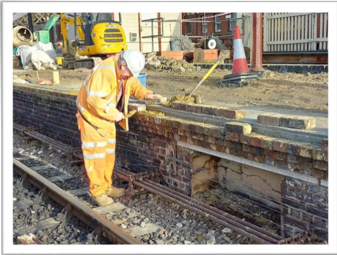
Bob the Builder replacing corbel brickwork. Photo: Jon Goff
