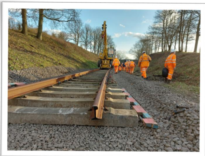
Left: Track laying at Vaux End. Photo: Jon Goff
