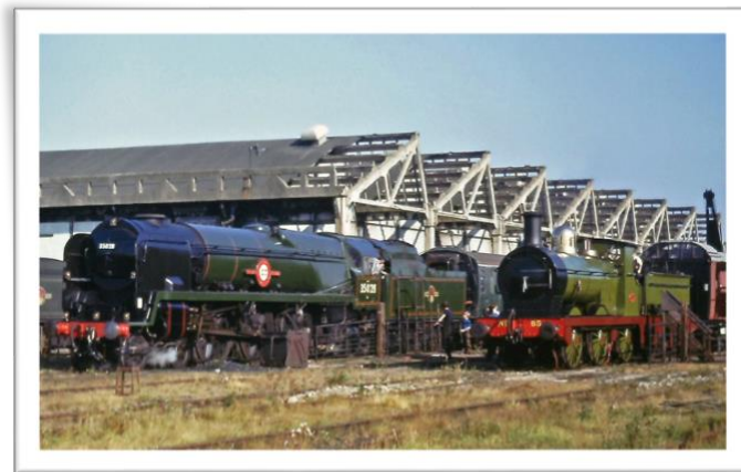
Top to bottom: Now in Ashford Shed – 17 July 1966 Photo: Keith Sturt
