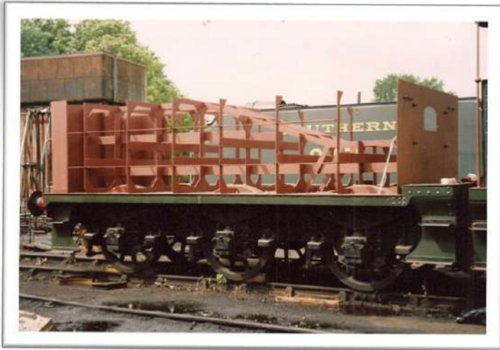
Tender tank under construction
