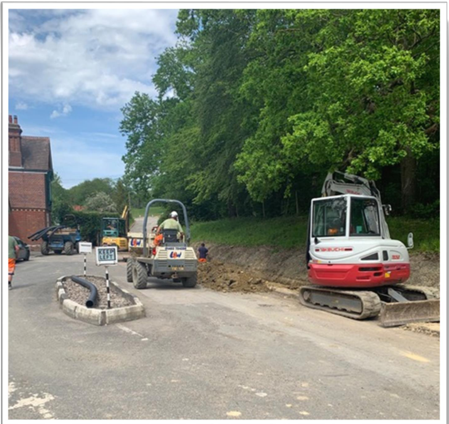
Installing the ducting.
