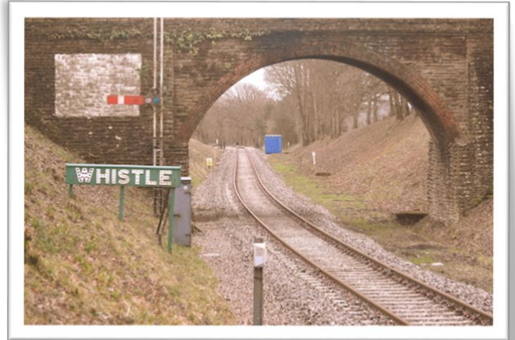
Looking south towards Horsted Keynes from Horsted House Farm Bridge with replacement track Photo: Jon Goff
