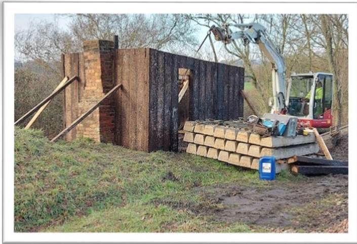
Vaux End hut being rebuilt around the old chimney
