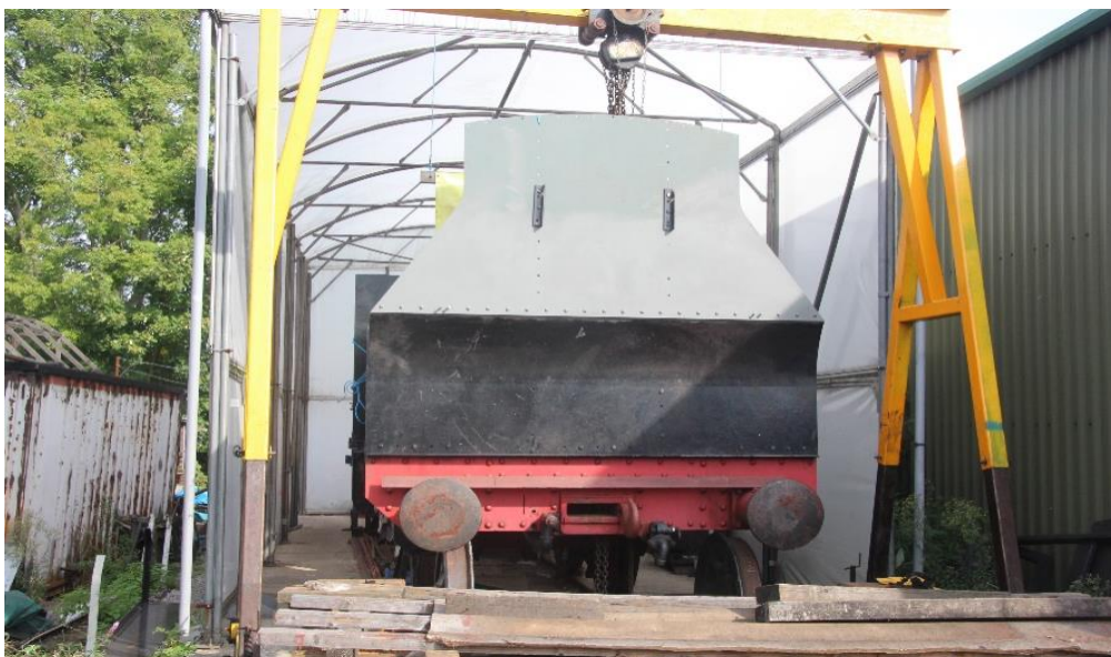
Rear Bunker Panel in it's Final Position and Bolted Down to the Underframe
