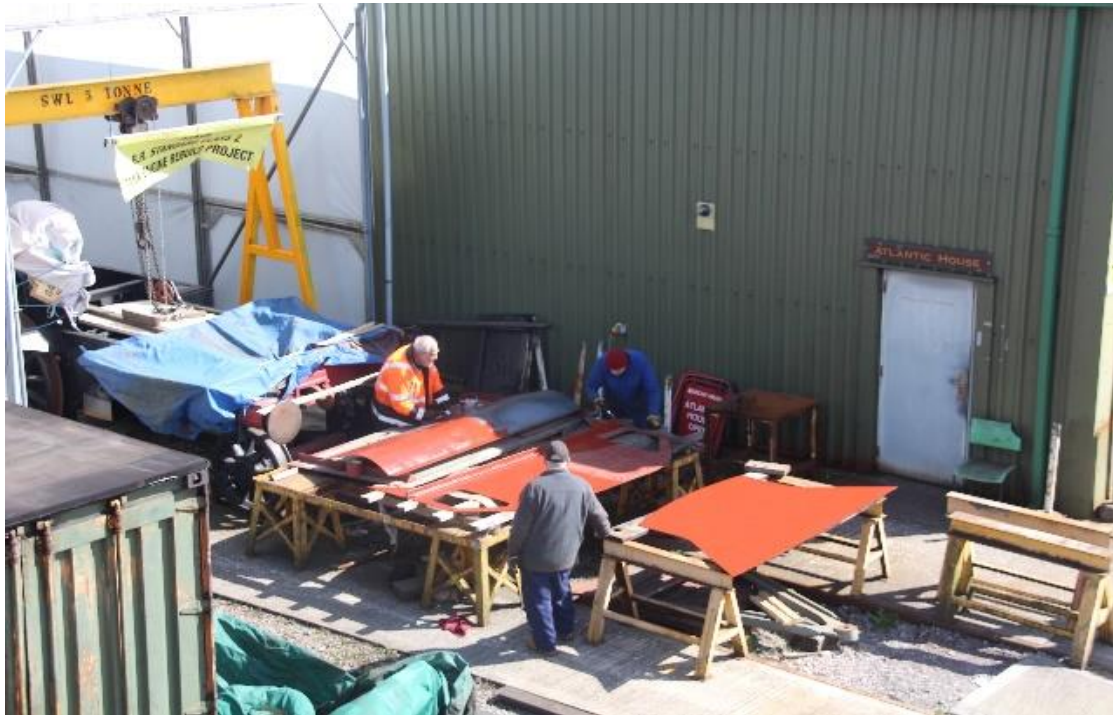
Front and Rear Bunker Panels and the Refurbished Gantry
